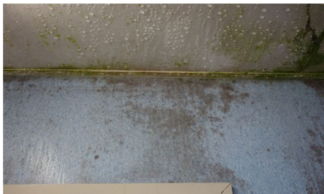
Mould on the ceiling and wall of a minimum security wing bathroom
