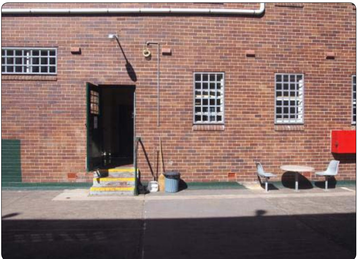
Stair access to the yard from an accommodation area at MSPC 3.
