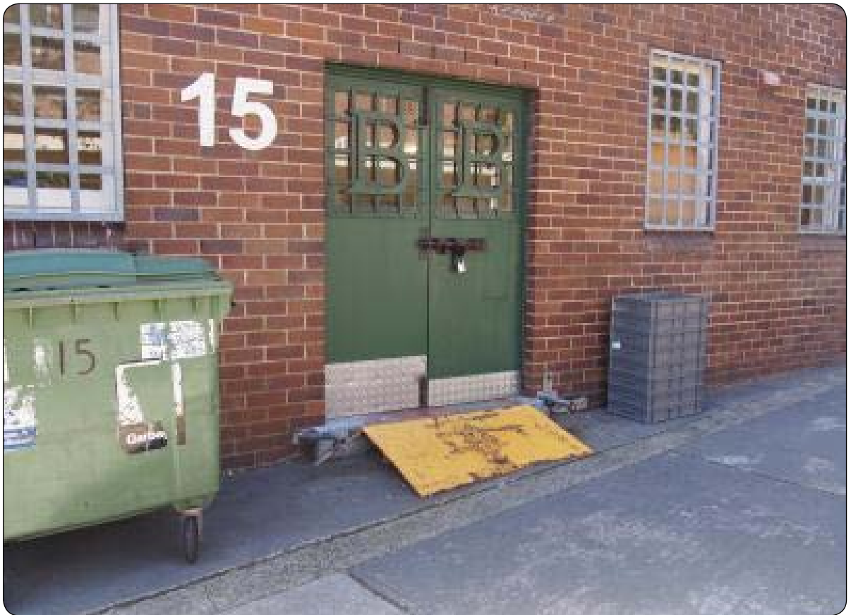
An improvised ramp from an accommodation area to allow access to the clinic at MSPC 3.
