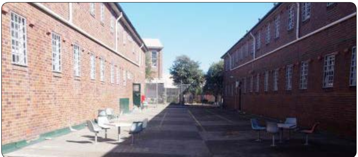
An accommodation area yard at MSPC 3: there is no shelter or appropriate seating.
