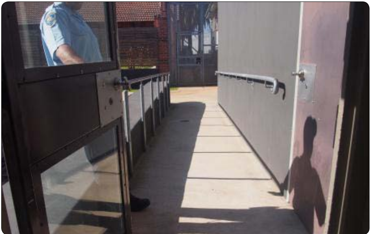
Sloped pathways at SWCC, railings and wide door entries.
