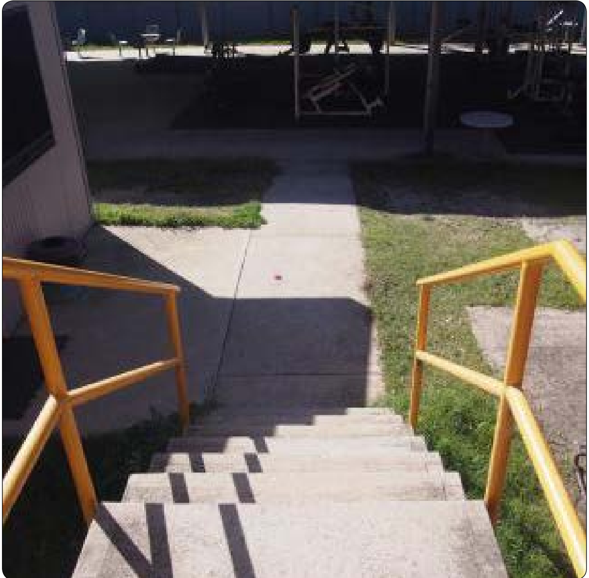
The oval and exercise equipment must be accessed via stairs at MSPC 3.
