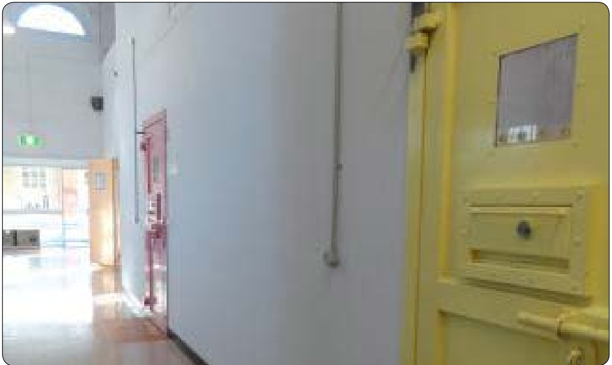
Colour-coded cell doors at KWU for assisting inmates with memory loss and vision impairment.
