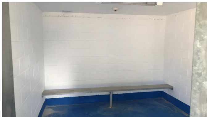
Reception area - external holding cell
