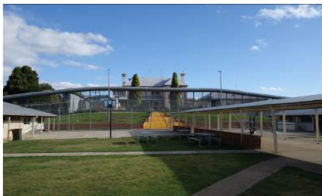
Main accommodation area
