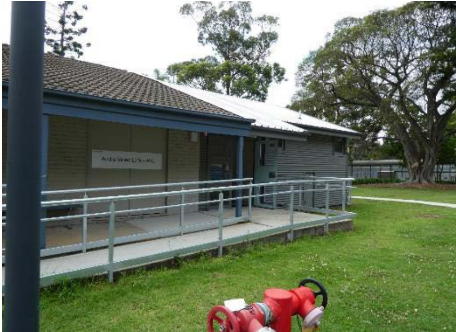
AVL facility, external view
