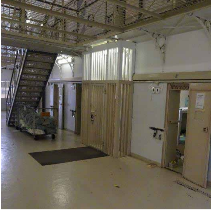
Maximum security unit corridor with stairs to the upper landing
