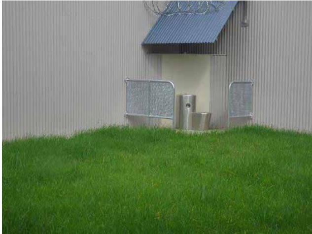
View of exercise yard toilet from the corridor
